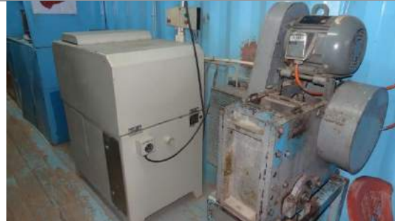
B Crusher and pulveriser
