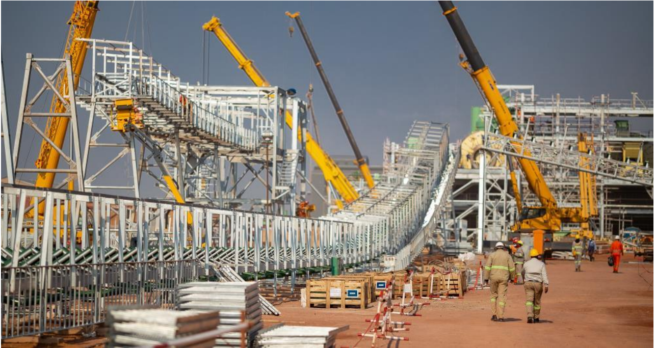
Cranes lifting sections of the Phase 2 ore conveyors into place.
