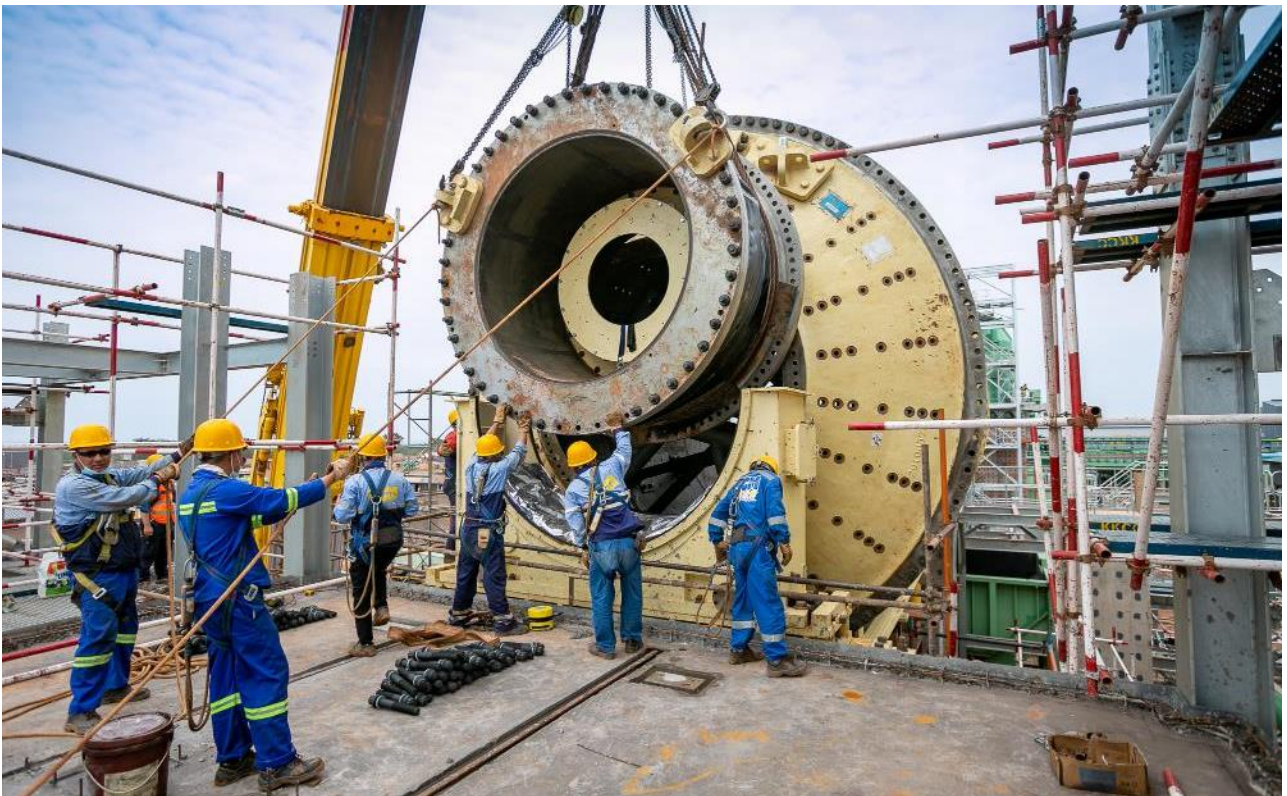
Installing the trunion bearing on the Phase 2 primary ball mill.
