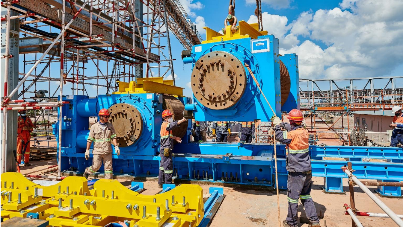
The Phase 2 HPGR being lifted into place.
