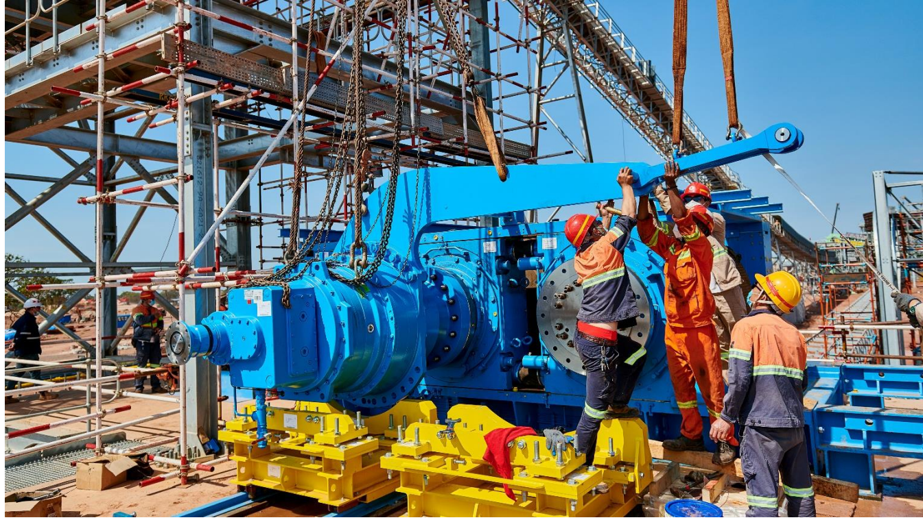
One of two Phase 2 HPGR motors being lifted into place.
