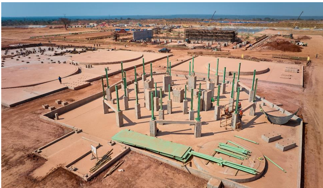
Photo: Construction of the concentrate thickener base is progressing well at Kamo-Kakula's Phase 3 concentrator site.
