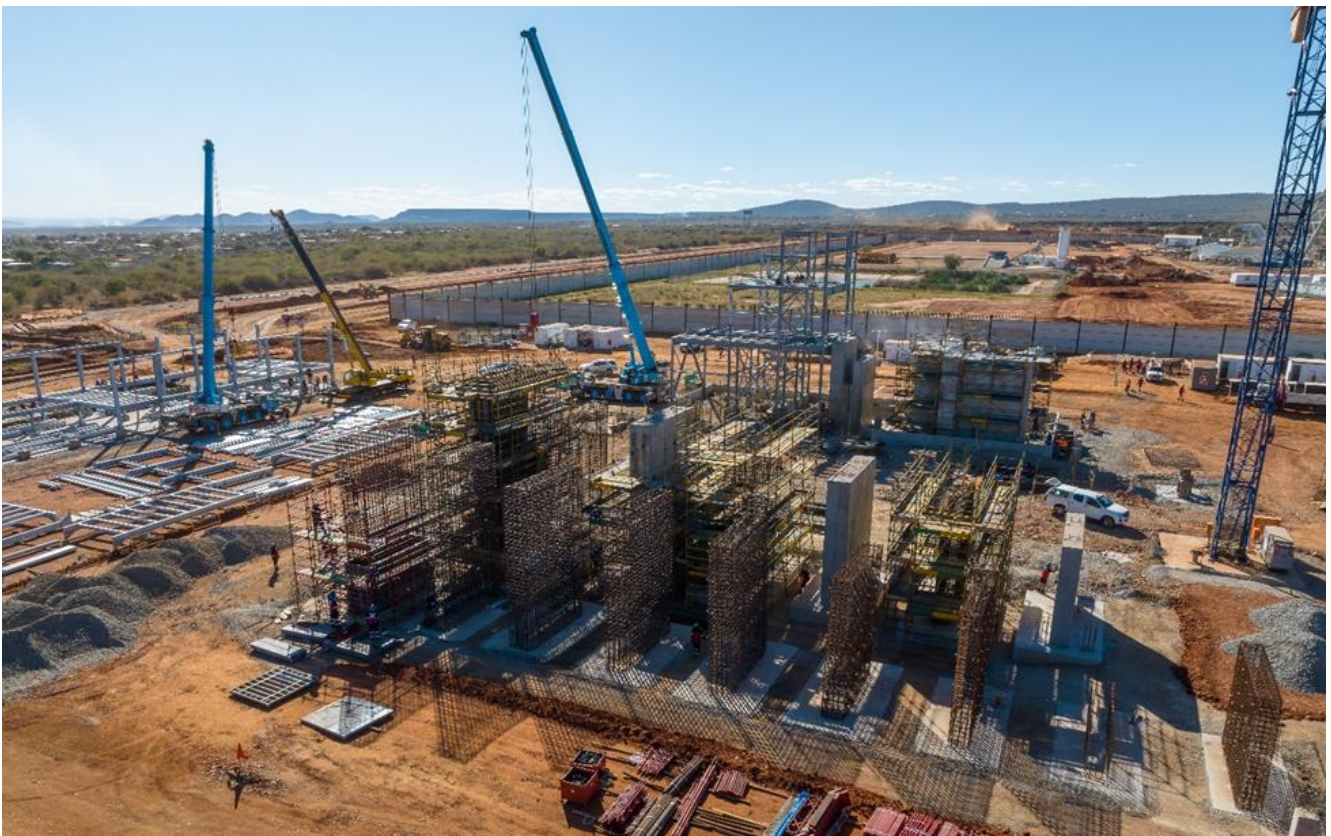
Photo: Foundation for Platreef's Phase 1 flotation cells is advancing well. Platreef's Phase 1 concentrator is on schedule for first production in Q3 2024, with all foundation concrete poured.
