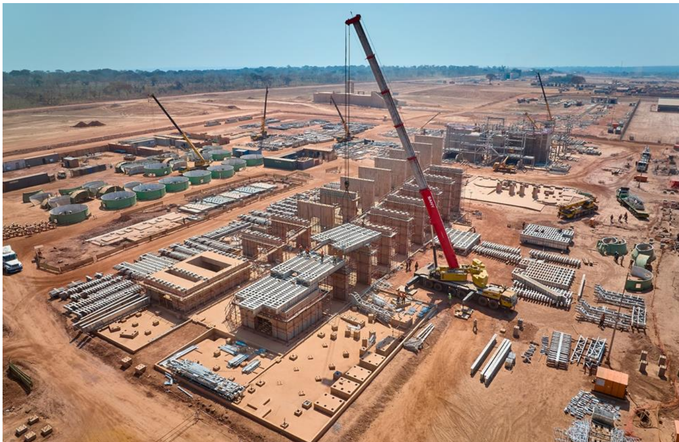
Photo: Construction of the concentrate thickener base is progressing well at Kamo-Kakula's Phase 3 concentrator site.
