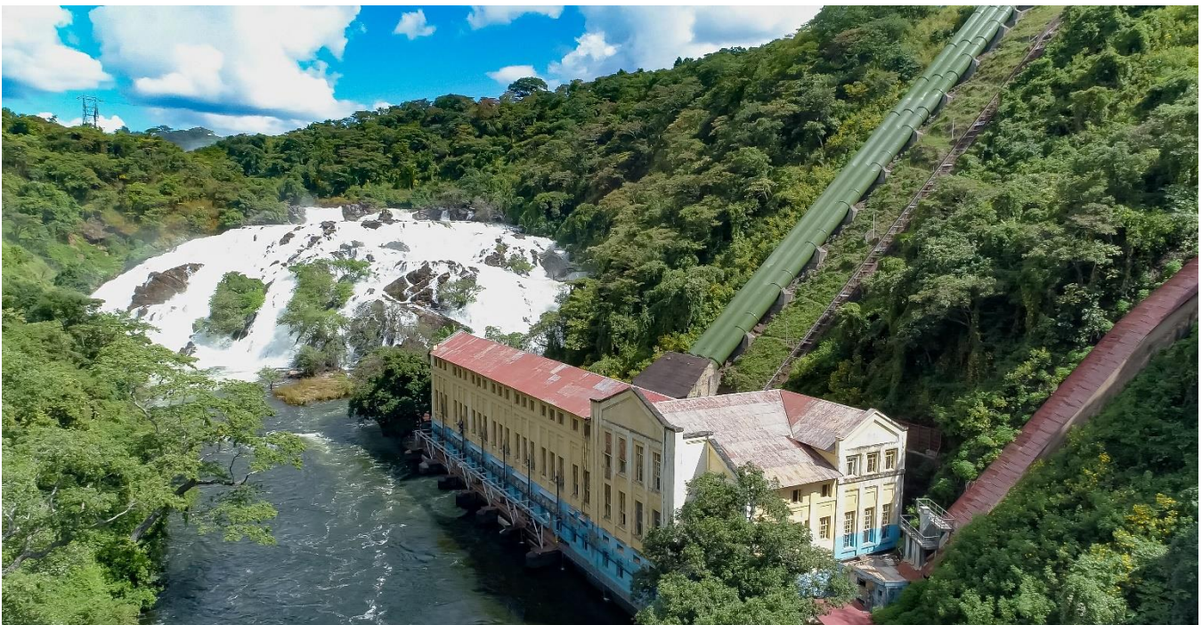
The hydropower building at Mwadingusha and the green penstocks that funnel water from the dam to drive the six new turbines.
