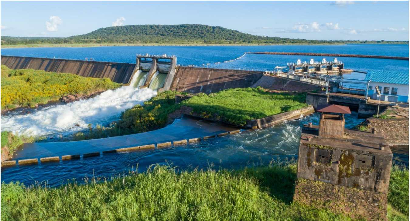
The Mwadingusha hydro dam, upstream from the hydropower building.
