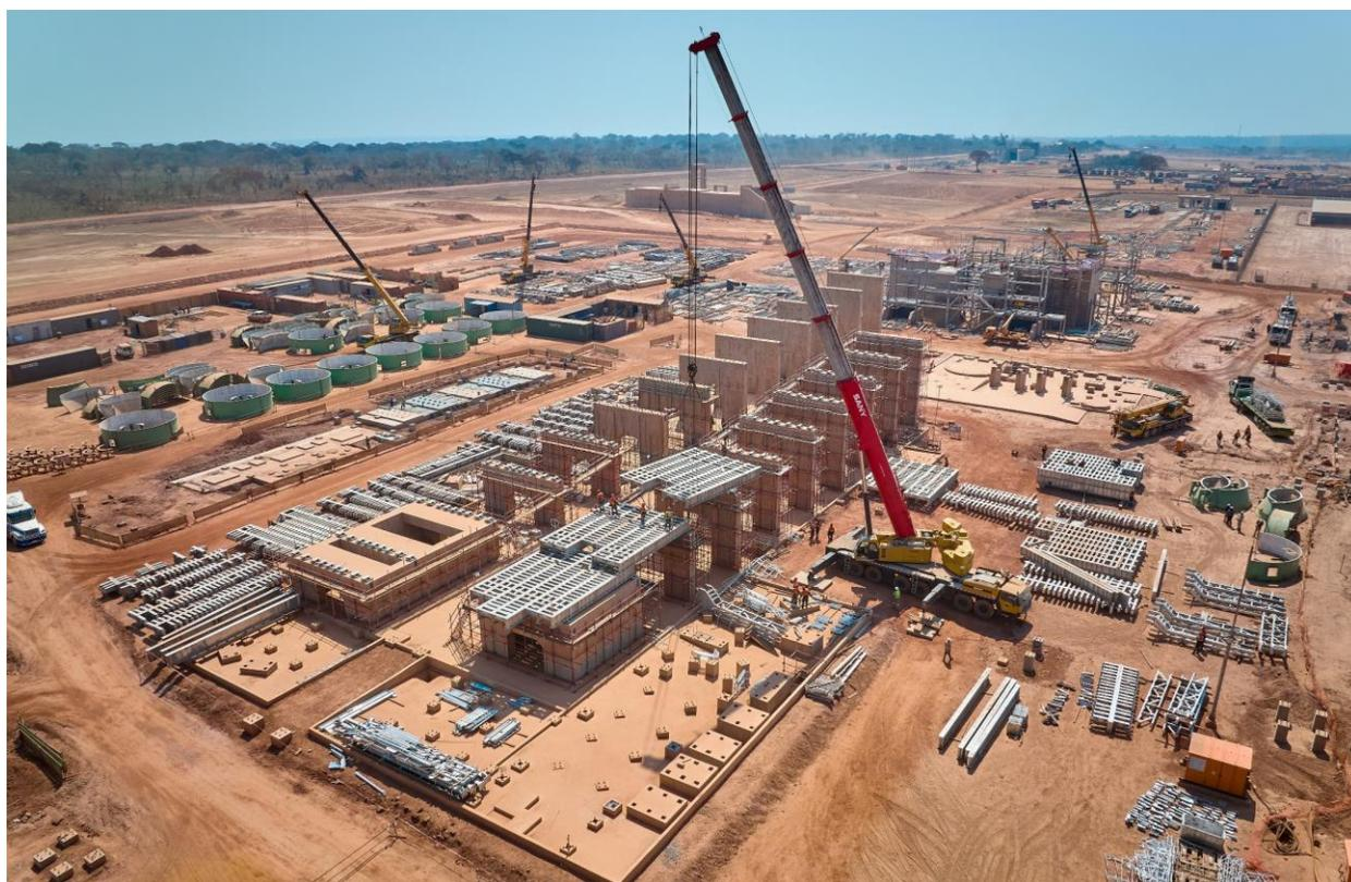
**Construction of the concentrate thickener base is progressing well at Kamo-Kakula's Phase 3 concentrator site.**
